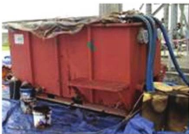
INSTALL TANK FOR COLLECTING LIQUID
